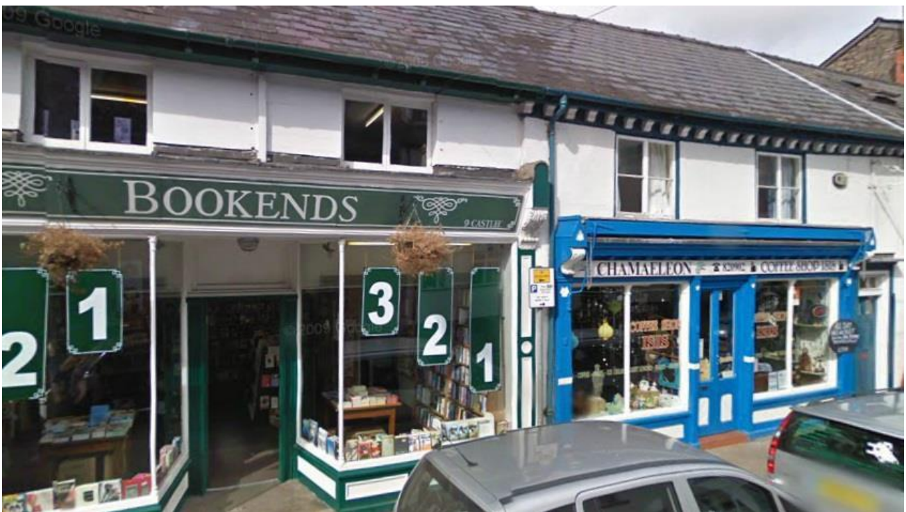
Traditional shop fronts in Castle Street
