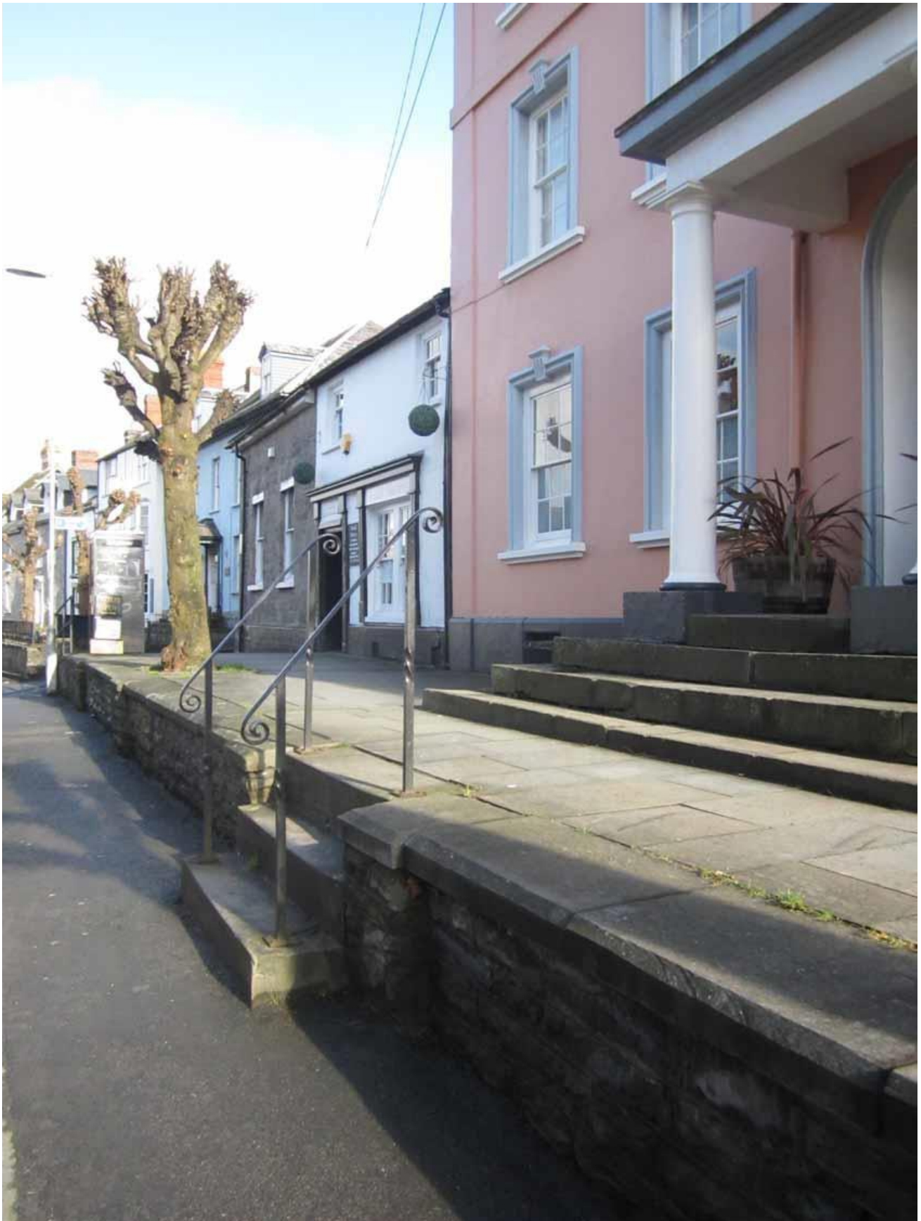
In Broad Street, the low retaining wall and natural stone paving on the raised pavement above are augmented by metal railings which help reinforce the steps between the two levels
